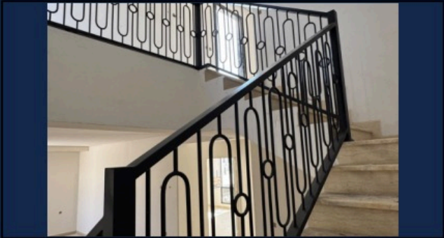
ALFANAR - ALFURSAN PROJECT UNDER NHC Installed stair handrails
